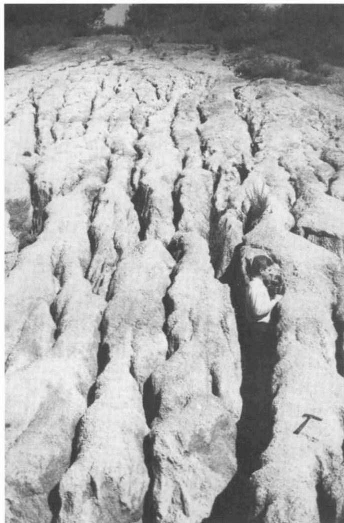
Fig. 11. Deep narrow gullies eroded in weathered granite or grus exposed in a road cutting near Cape Town, South Africa.
