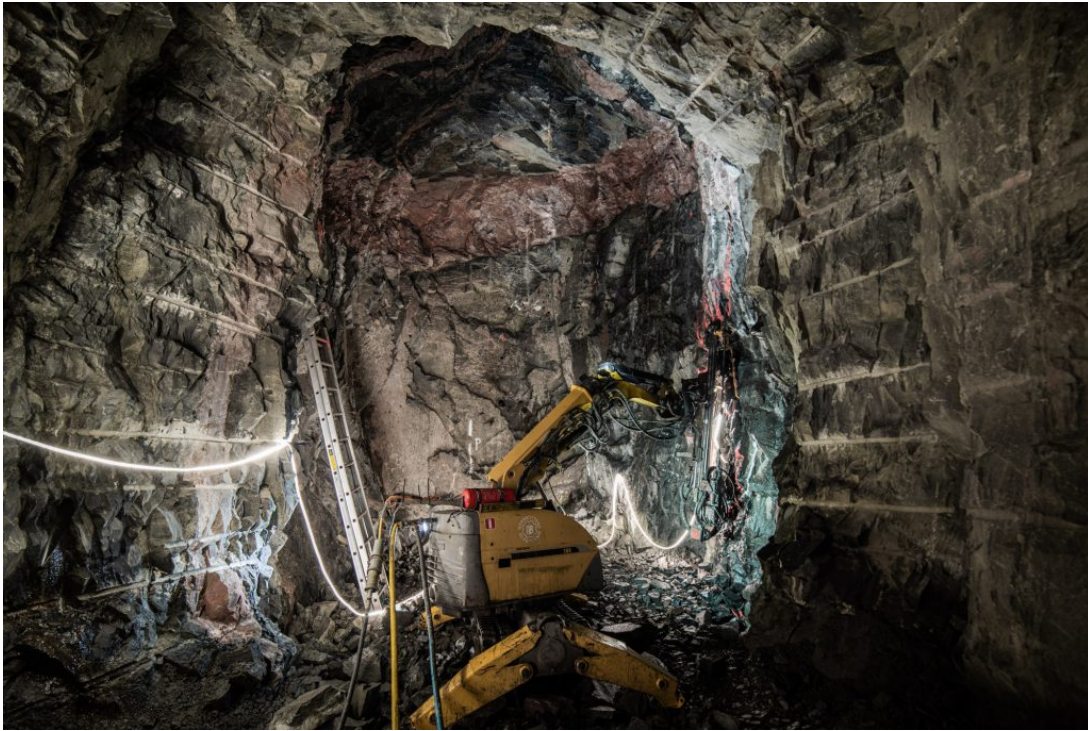
Figure 1.5: Rock cavern in Skallen (Sweden). Source: PV Magazine
