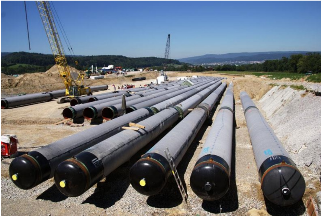
Figure 1.6: Pipe storage construction working. Source: Zürich Transport AG
