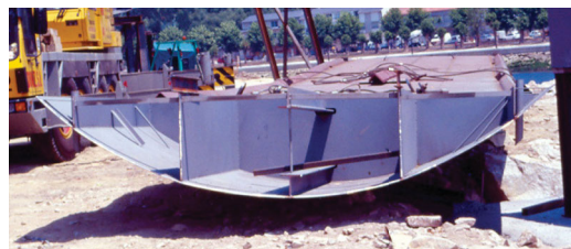
(b) Deck cross-section with circular segment shape.
