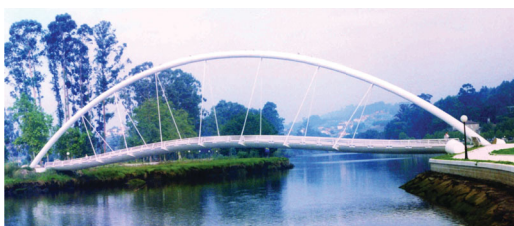
(a) General view of the footbridge.
