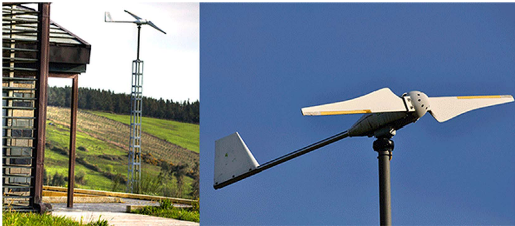
FIGURE 4. Low power wind turbine installed in Sotavento bioclimatic house.
