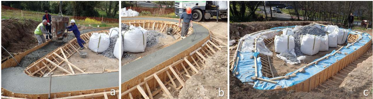
Figure 9. Placement, vibrating and curing of strip footing concretes (non-structural and structural).
