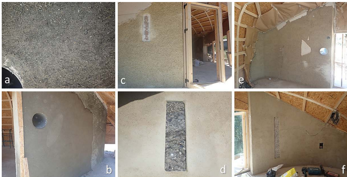
Figure 16. Coating mortars applied in the building: cement mortars (left), lime mortars (middle), and clay mortars (right).
