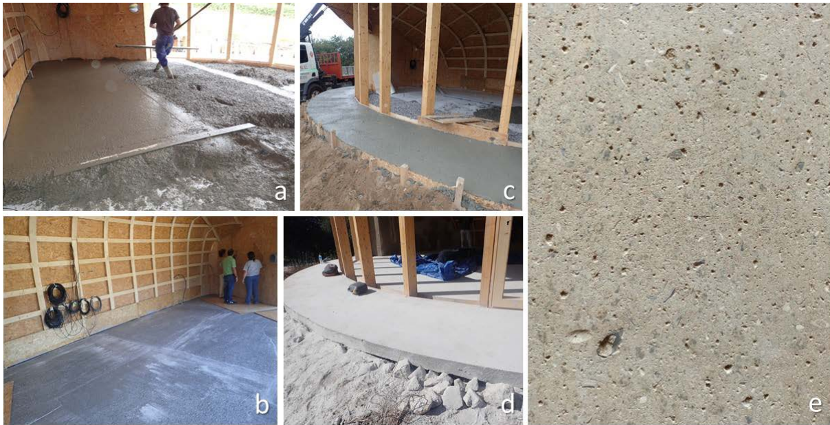
Figure 10. Construction process of the concrete slab and the structural piece.
