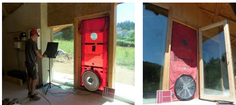
Figure 19. Blower door test carried out in the experimental building.
