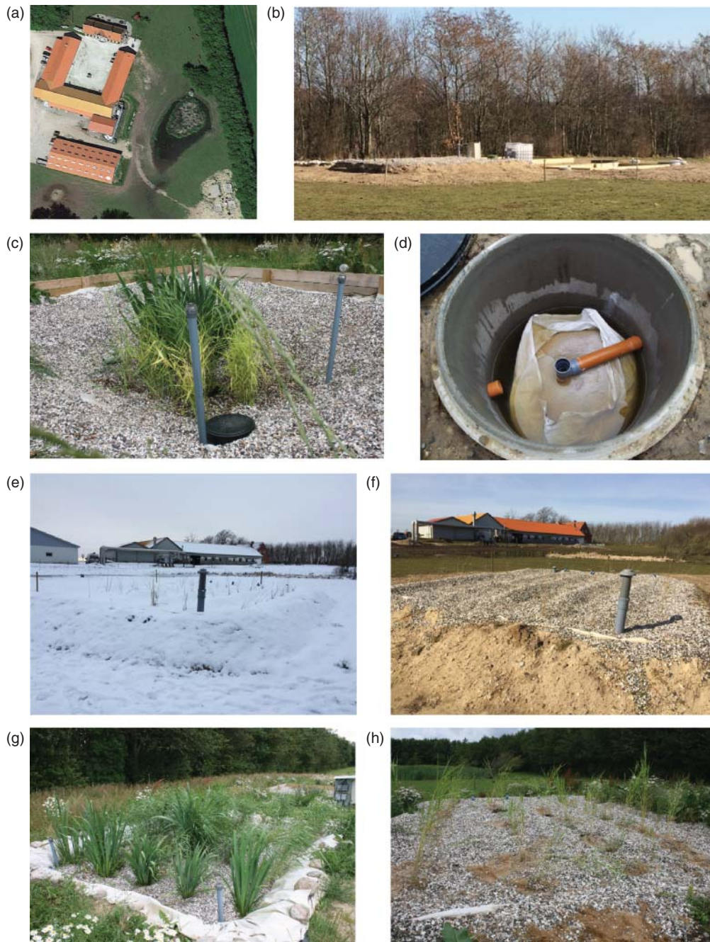
Figure 3.2 Satellite image showing the location of the treatment plant (a); a general view of the plant once it was established (b); details of HF bed (c); detail of P removal unit (d); state of the system during Campaign 1 at winter 2015 (e); state of the non-aerated VF bed during Campaign 2 (f); the two VF beds during Campaign 3 (aerated VF bed: g; passively aerated VF bed: h).
