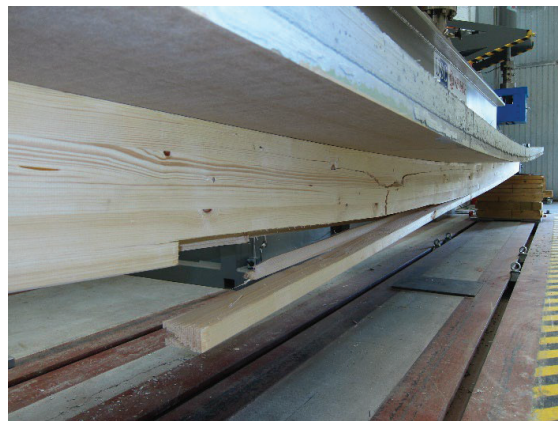
Figure 6: Tensile failure in the lower fibre of the timber joist.
