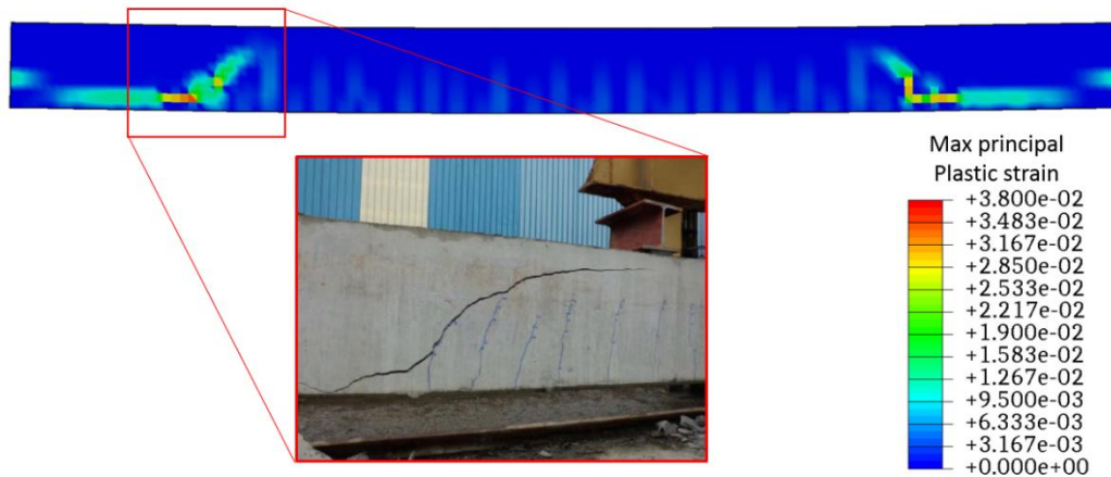
387 388 Figure 10. Shear test of beam with concrete M0: FEA model with principal plastic strain after a deflection 389 of 25.4 mm and detail photography of cracking pattern on one extreme of the beam at shear failure 390
