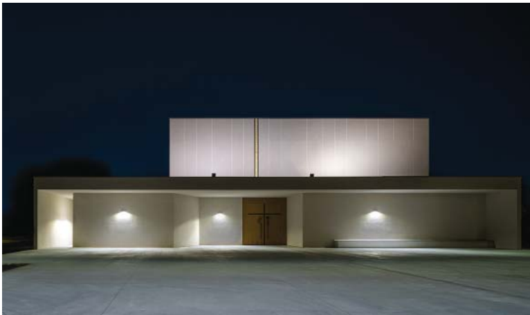
Fig. 02. External view. Fig. 03. Liturgical hall.
