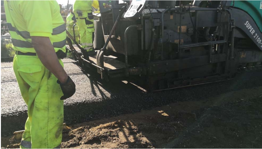
Figure 11. Construction of the base layer of GE-1 manufactured with ‘eNanocel-07’.
