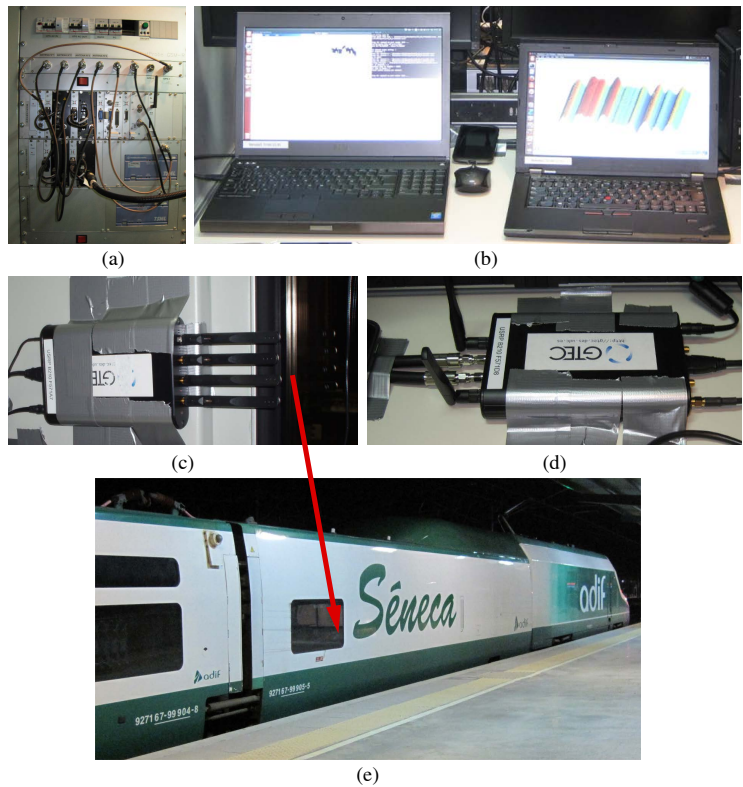
Figure 3: LTE testbed receiver installed at the train carriage: (a) connection panel for the external antennas; (b) laptops of both testbed receiver nodes; (c) receiver node with its own indoor antennas (only two are used); (d) receiver node connected to the outdoor antennas (the additional attached antennas are just meant for test purposes); and (e) placement of the indoor antennas in the train carriage.
