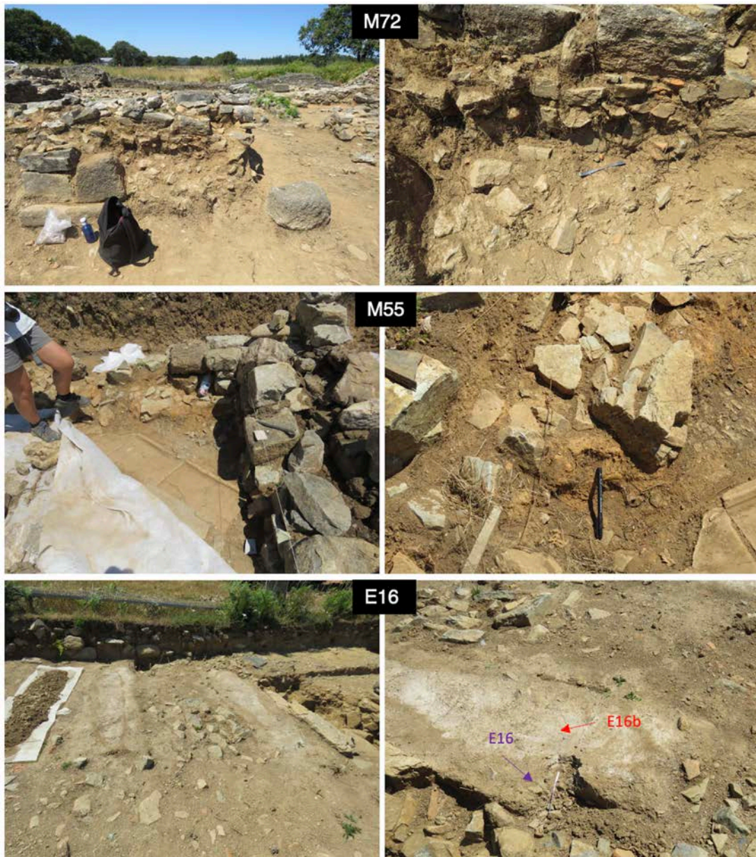
Figure 2b (cont.): Location and detail of mortar samples of joints M72 and M55 and pavement E16. The tip of the spatula identifies the sampling point. A detail of the surface of pavement E16 is also shown, which makes it possible to distinguish the more whitish color that affects the most superficial 2 cm (where sample E16b was collected) in contrast to the rest of the pavement, which has a more reddish color.
