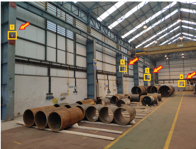
Figure 2: Test scenario (left side of the workshop) with the anchors (inside yellow squares).
