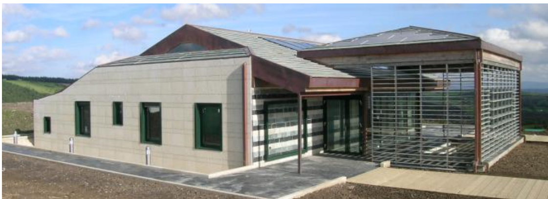
Figure 1. Sotavento bioclimatic house.
