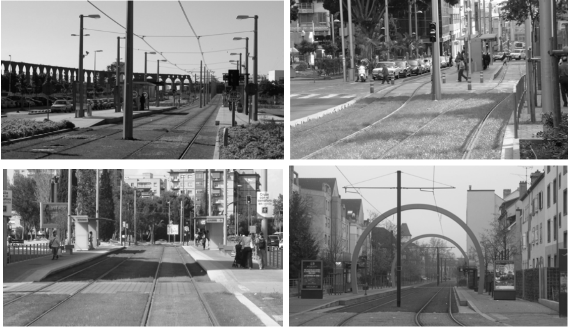
FIGURE 8 Stop treatment in turf track. a) Turf track interruption at stop in Porto (Portugal); b) Turf track interruption at stop in Tenerife (Spain); c) Turf track through stop in Zaragoza (Spain); d) Turf track through stop in Mulhouse (France).
