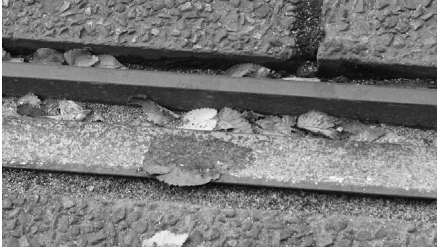
FIGURE 7 Leaves stuck to rail head.
