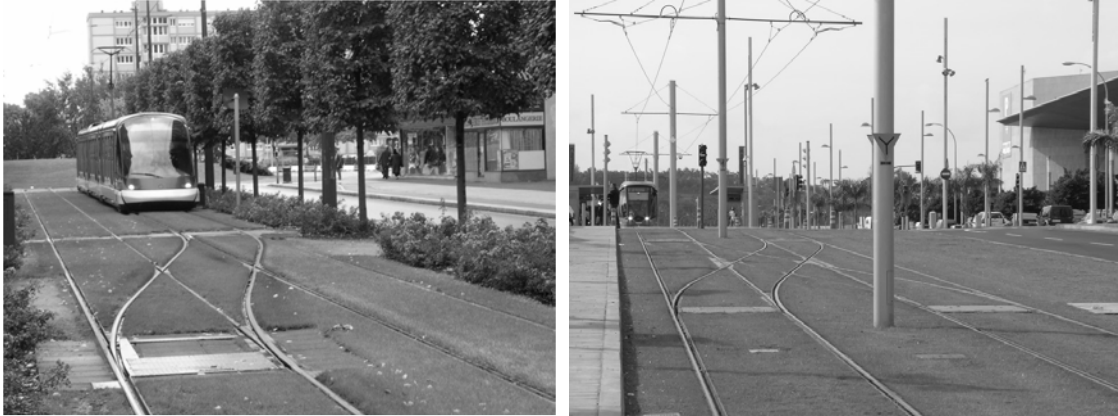
FIGURE 6 Turnouts and crossings in turf track. a) Strasbourg (France); b) Tenerife (Spain).
