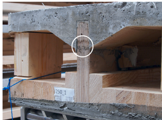
Fig. 12. Slippage of the connection in the 250.1-C test.
