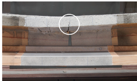
Fig. 9. Cracking in the concrete slab. Test 350.1-C.
