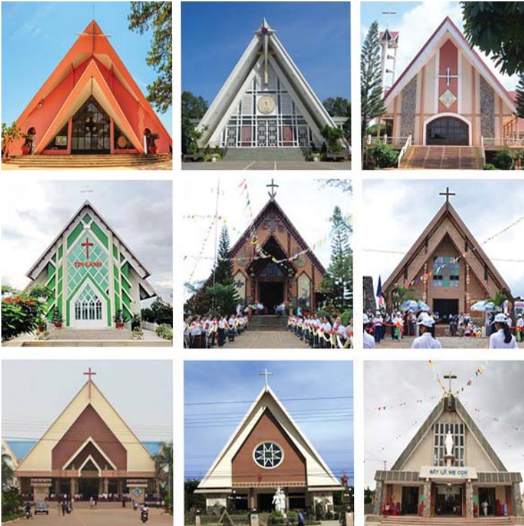
Fig. 17. Church design as mass-copied. Fig. 18. Nguyen Thanh Ho (contractor), Cam Ly parish church, Lam Dong (Vietnam), 1960-68. Fig. 19. Some churches in Lam Dong and Dong Nai; mass-copied and modify to many new versions.
