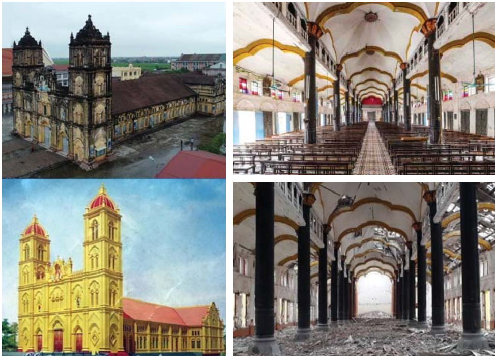
Fig. 20. Bui Chu Cathedral (Vietnam); demolished on 2020, July 20.
