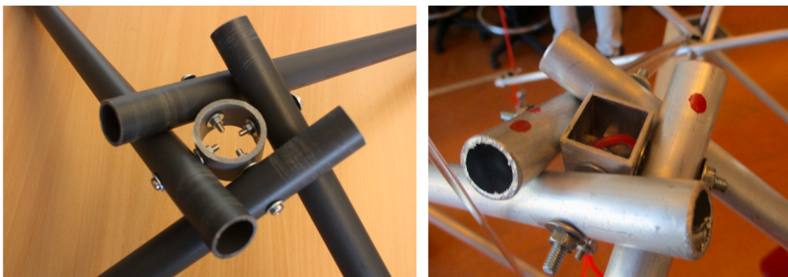
Fig. 3. Reciprocal linkages. Circular and square section.
