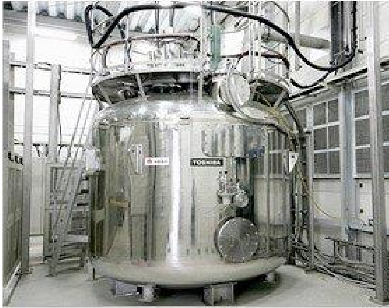
Figure 34. One of the world's largest SMES magnetic storage tanks in Kameyama, Japan.
