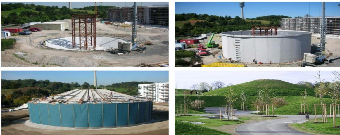
Figure 19. Construction of Seasonal Heat Storage in Munich, 5700 \text{ m}^3 , 2007.
