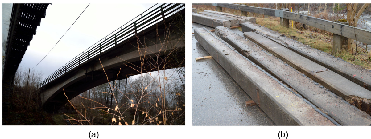
Figure 1. Overview of Gullspång bridge (a) and extracted edge beams (b).
