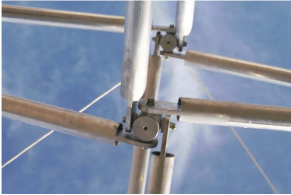
Figure 5.- Articulated linkages.
