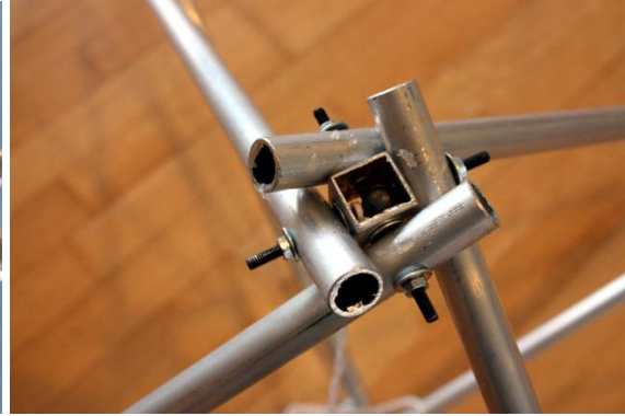
Figure 6.- Reciprocal linkage.
