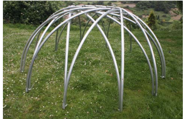
Figure 20: Prototype of a vertical axis dome.
