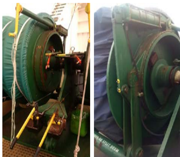
Figure 8. LNG Tanker "British Innovator": Band brake spring-applied and hydraulically release by hydraulic hand pump.
