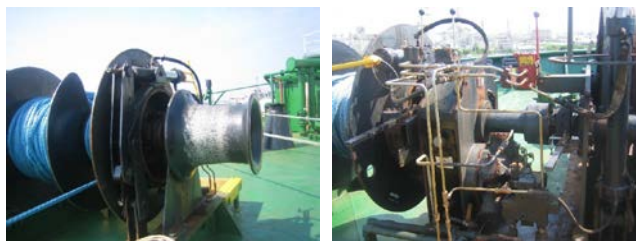
Figure 9. Tanker "Florida Voyager": Band brake spring-applied and hydraulically released by taking advantage of the main hydraulic pressure on winches with hydraulic drives.
