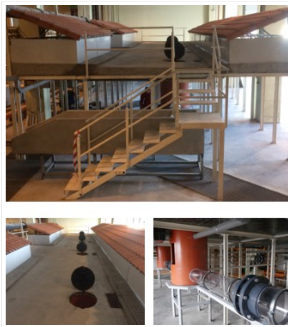
Figure 4. PCEHU main general view (above) and physical model surface and drainage system (below).
