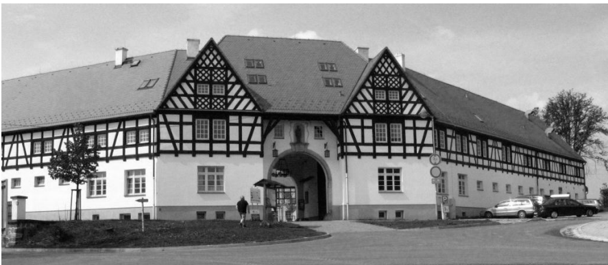
Figure 4. Bernard’s grange (Source: IOER)
