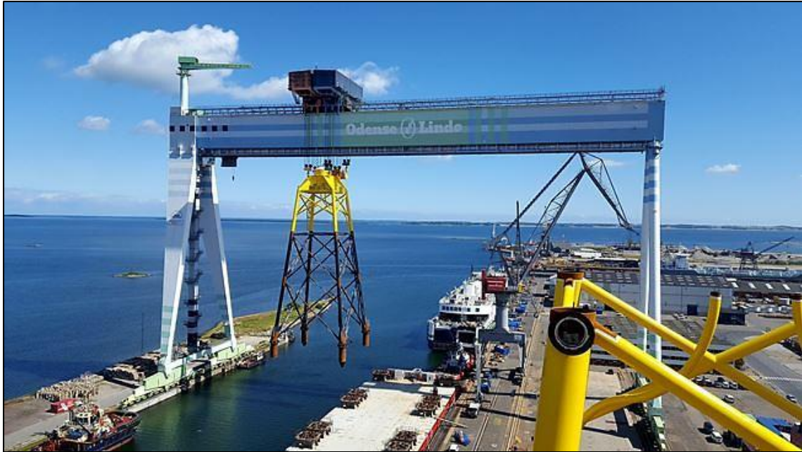
Figura 28. Load Out jackets Wikinger Astillero Bladt Industries
