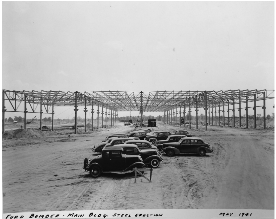
FORD BOMBER - MAIN BLDG. STEEL ERECTION
