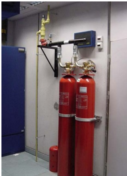
Figure 1.30: Extinction system with very small length of discharge's pipe.
