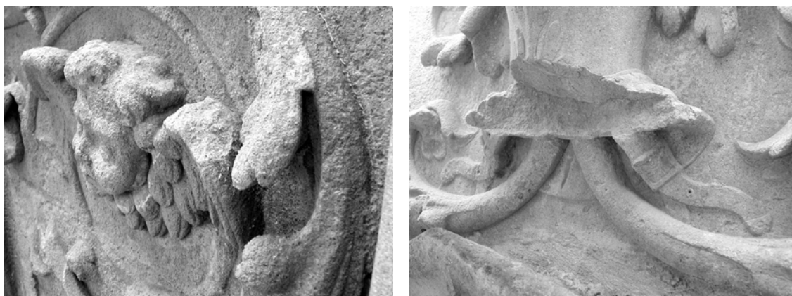
Figs. 6 and 7. Degradation of main facade in stone's sculptural iconography
