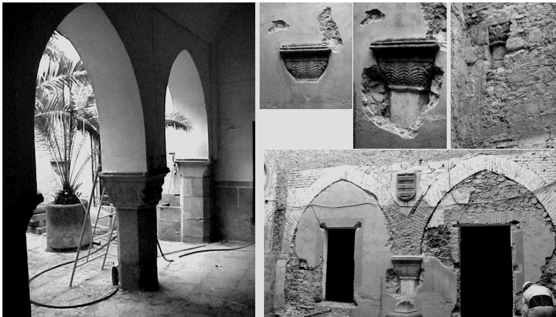
Fig. 9. Arches, in the central courtyard. In two columns appeared, with vegetable reliefs in their capitals that were evidence of a higher corridor.
