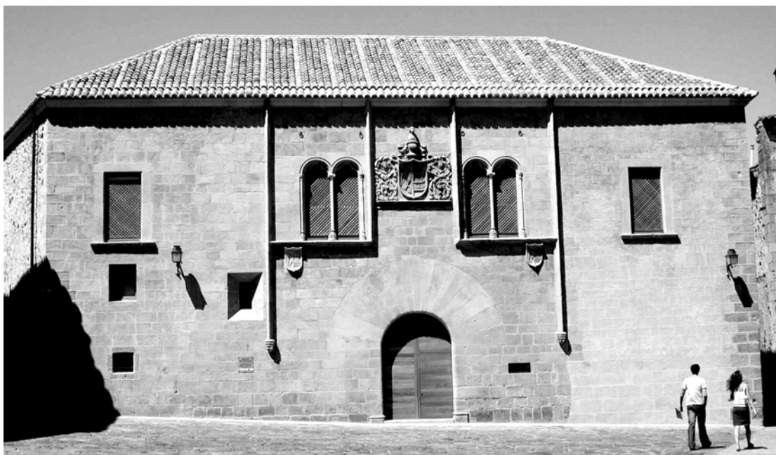
Fig. 3. Palace of Mayoralgo after restoration (2005).
