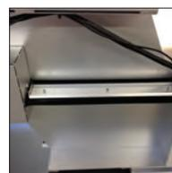
The automatic bypass damper makes the outdoor air bypass the heat exchanger when heat recovery is not required, thereby saving energy.
