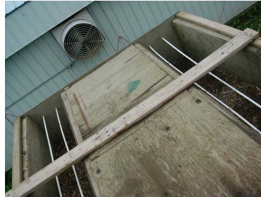
Figure 6. The side walls of a biofilter held with a plank
