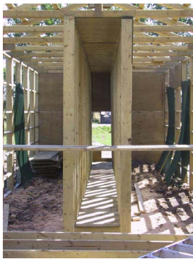
Figure 4a. Horizontal airflow biofilter (end view).
