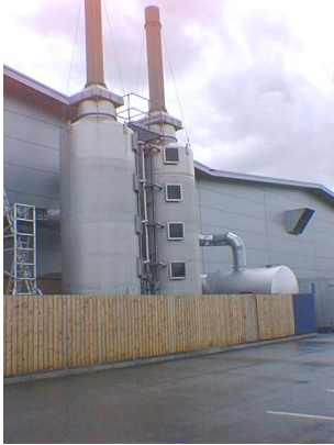
Figure 1. Biotrickling filter for DCM abatement, Senior Aerospace, UK. 2 \times 20,000 \text{ m}^3/\text{h} , 4 s contact time.
