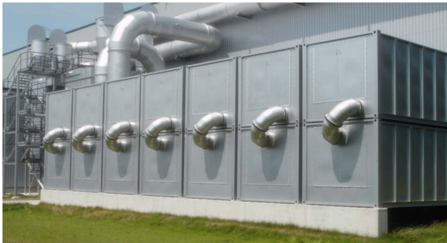
Figure 6. Municipal waste treatment; Multi-Stage Biofilter, Airflow 80.000 m 3 /h.
