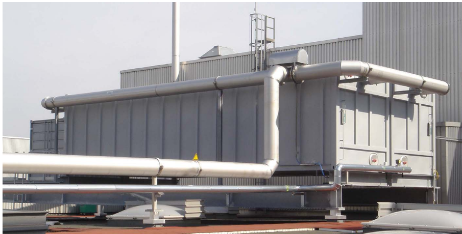
Figure 7. BMW AG. Multi-Stage Biofilter, Airflow 6.000 m 3 /h.
