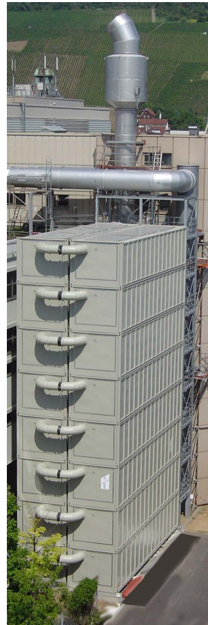
Figure 4. DaimlerChrysler; Multi-Stage Biofilter, Airflow 100.000 m 3 /h.
