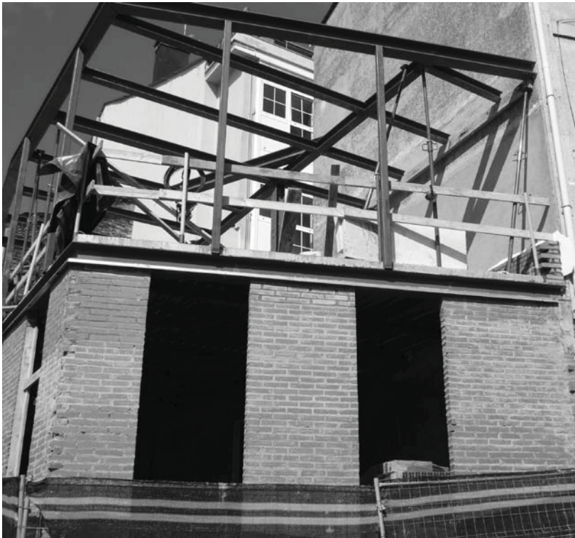
Figure 6. Housing in Rúa Falcón under construction.
