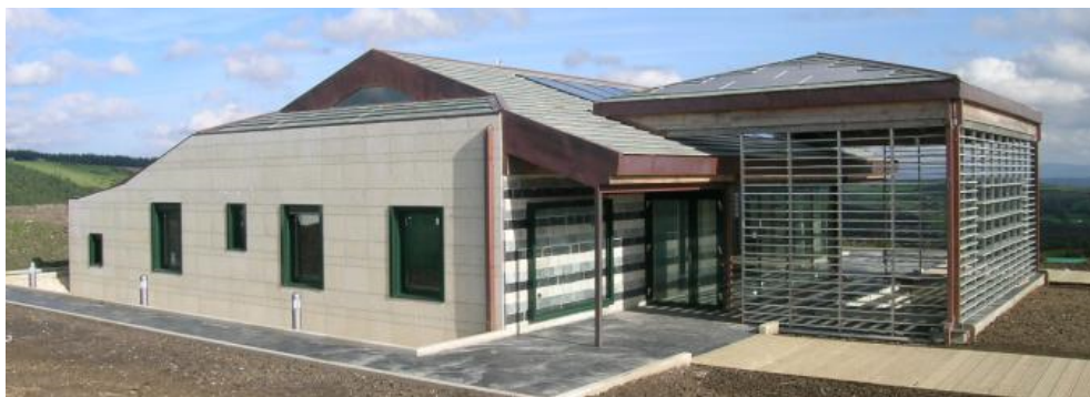
Figure 1: External view of the bioclimatic house
