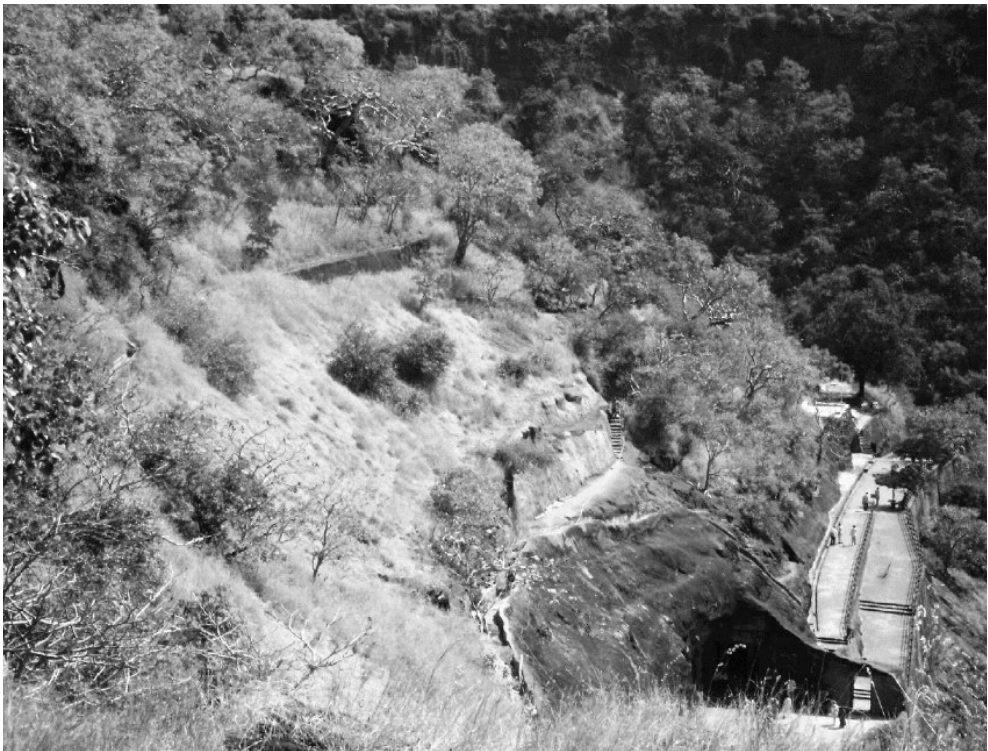
Fig. 4. Structure erected for slope protection at the Ajanta Caves World Heritage Site. It is designed “ideally” to avoid distraction of visitors’ attention from the site itself, this structure looks similarly to authentic natural (basalts) and artificial (caves) features.
