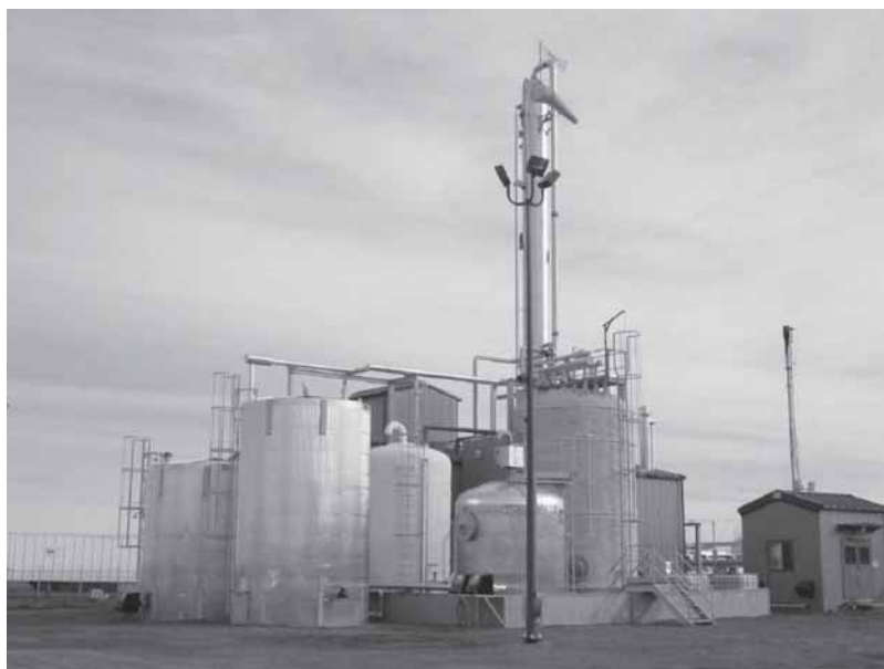
Figure 4. First commercial full-scale unit for biotechnological \text{H}_2\text{S} removal from high pressure natural gas. The Shell-Paques unit is designed to meet a \text{H}_2\text{S} specification of <4 ppm volume on the treated natural gas.
