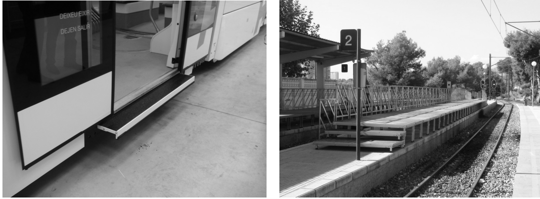
FIGURE 4 Passenger access issues: a) Retractable ramp of light rail vehicle being deployed in workshop; b) Provisional structure for level boarding in shared platforms between tram-trains and diesel trains.
