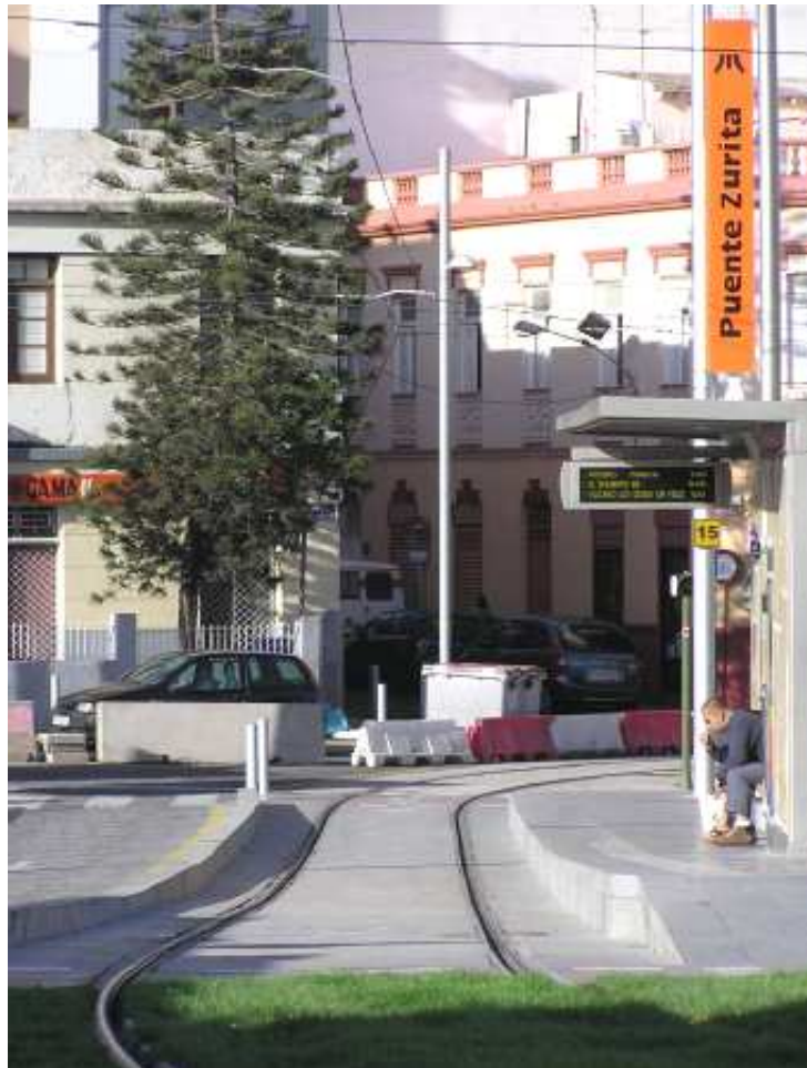
FIGURE 7 Station located in a sag vertical curve. Tenerife light rail. Source: (12)
