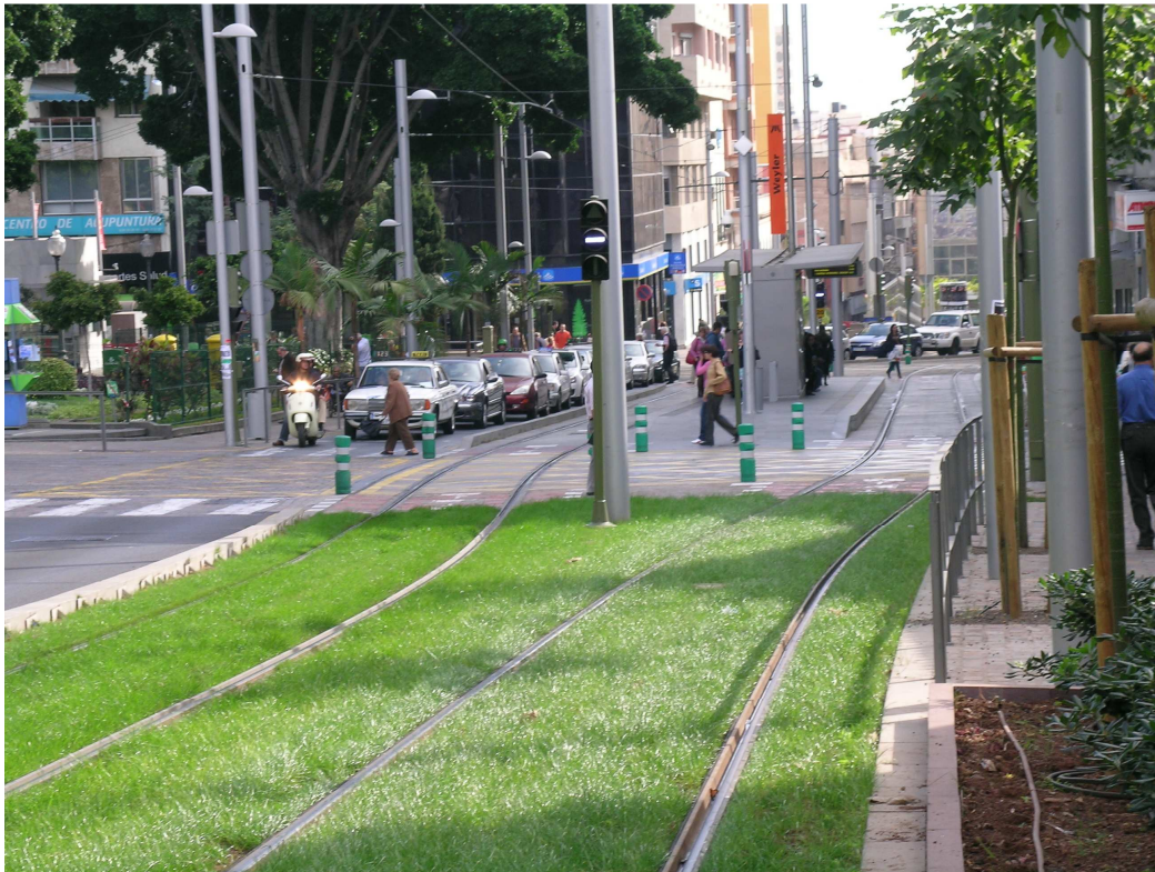
FIGURE 5 Station in which tangent tract is not extended to both sides of the platform. Tenerife light rail.
