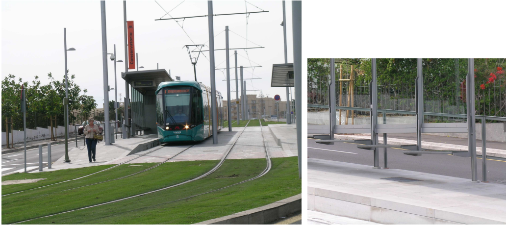
FIGURE 6 Vertical grade of 7.5% at station. See the detail of staggered seats in the shelter. Tenerife light rail.
