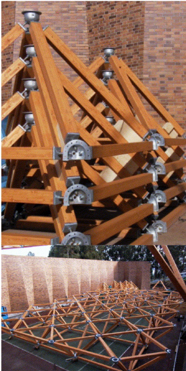
Fig. 2. Stacked space frame modules and view of stacked modules of the space frame before its assembling. Sports hall. Campus “A Zapateira”. A Coruña. Spain.
