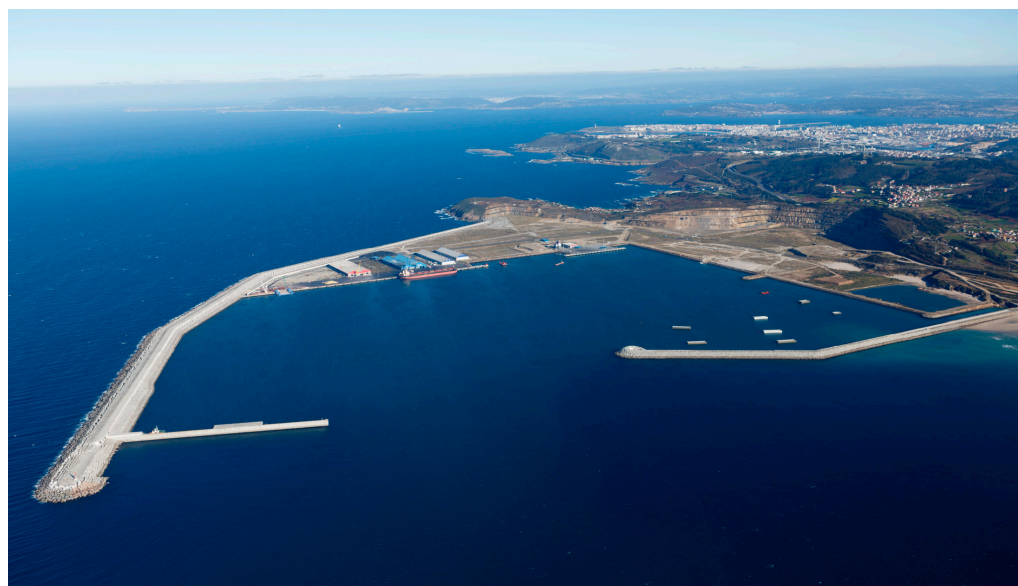
Figure 1. Aerial view of the outer port of Punta Langosteira, A Coruña, Spain.
