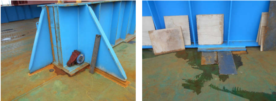
Figure 9. (a) Longitudinal and transverse brackets; (b) Thin metal ready to be placed below the central bearing plate.
