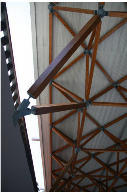
Figure 20: View of the timber spatial truss
