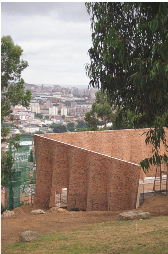
Figure 10: View of the brick walls
