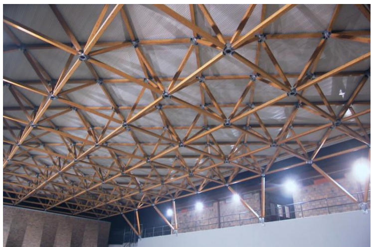
Figure 21: View of the timber spatial truss
