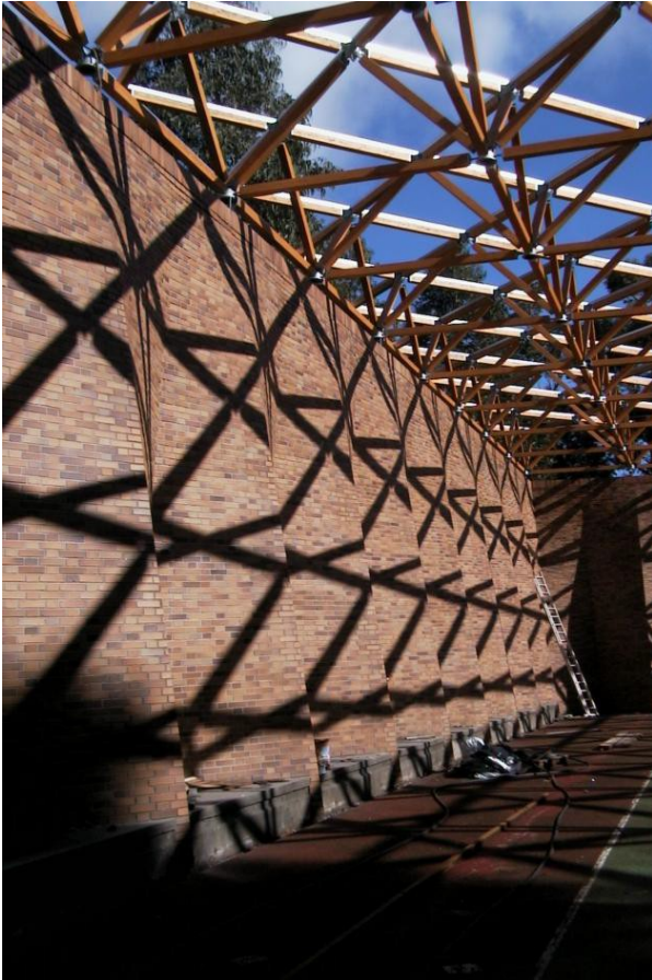
Figure 18: Internal view of the building
