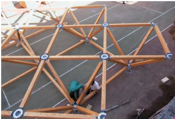
Figure 16: Assembly process of modules
