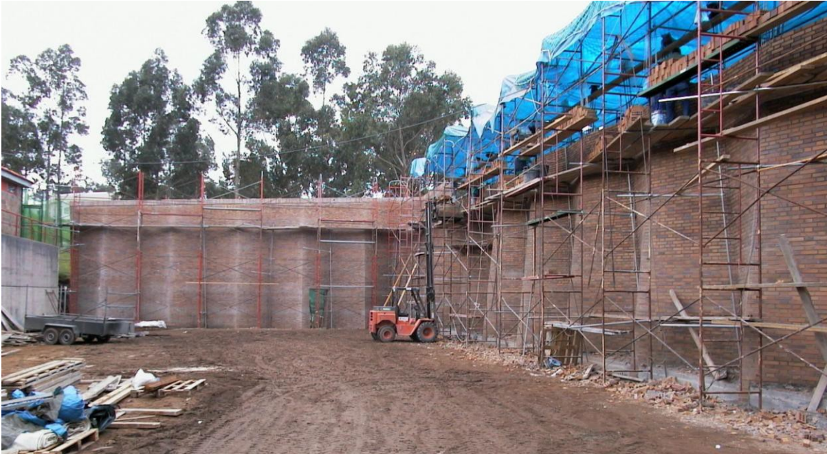
Figure 9: View of the brick walls
