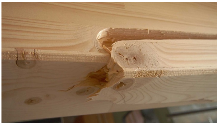
Fig. 10. Failure due to knots in the specimen F1/PIC-3.
