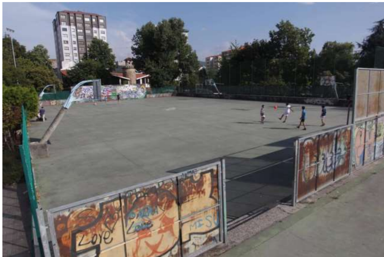
Covering and reaconditioning of the Campolongo public multisports courts at Pontevedra
