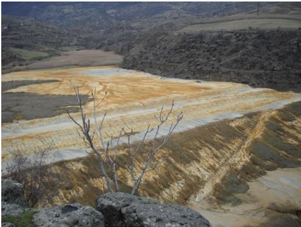
Figure 7. General view of Teghut tailing
