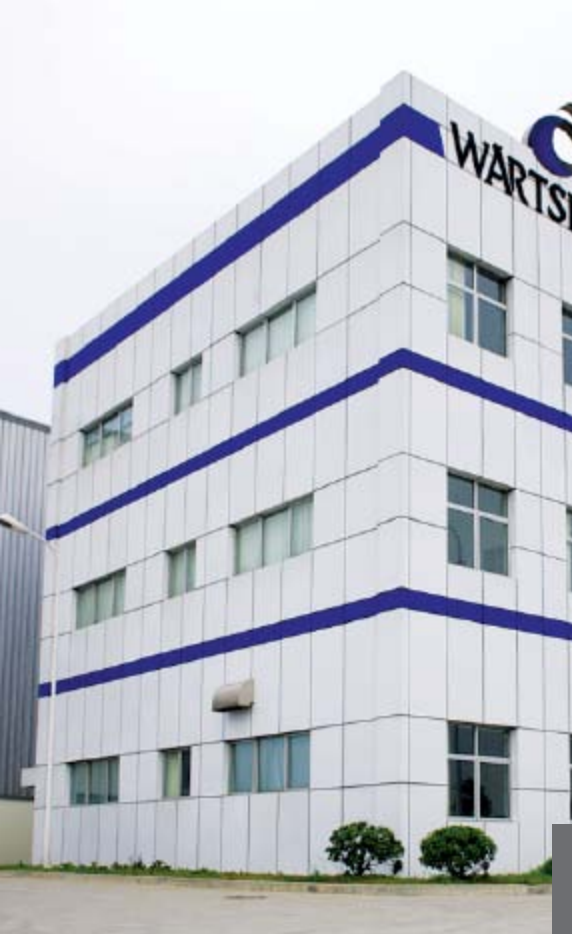
The Wärtsilä Plant in Wuxi, PR China, has produced transverse thrusters since end 2004.
