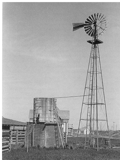
Fig. A.2.4: Rotor multipala [Gipe, 1993]
