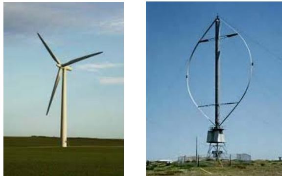
(a) Horizontal axis design. (b) Vertical axis design.
