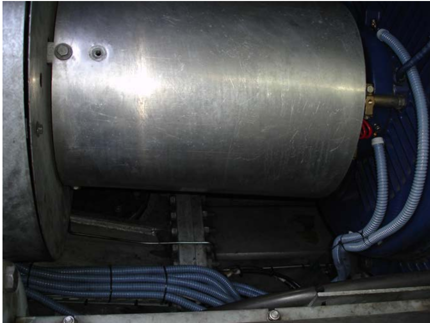
(a) Acceleration pick-ups installation.
