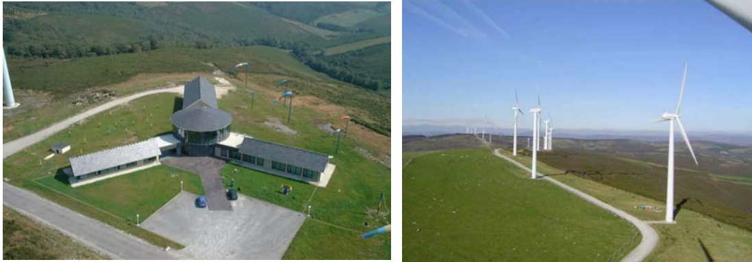
Figure 6.17: Sotavento's main control station and wind farm.
